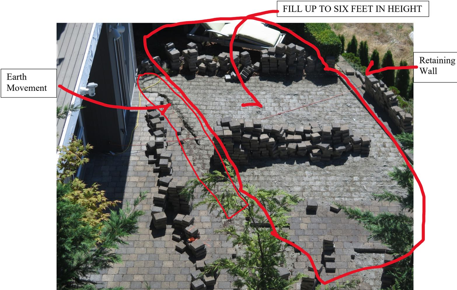
**7/22/2016 – RETAINING WALL, FILL, AND FAILED PAVING
