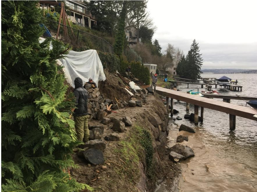
**02/02/2018 – EXCAVATION AND ROCKERY CONSTRUCTION IN SHORELINE SETBACK DURING BANNED SEASON WITH NO EROSION CONTROL,**
